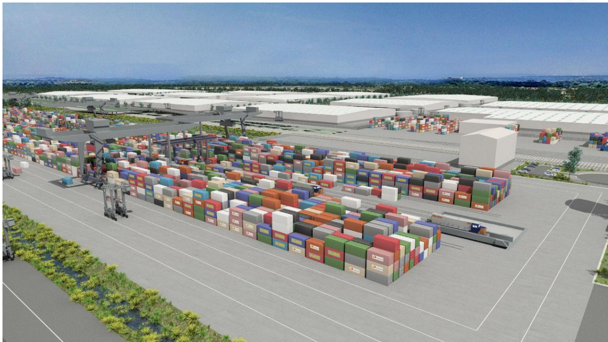
The IMEX terminal and some of the warehousing at the Moorebank intermodal freight precinct.
