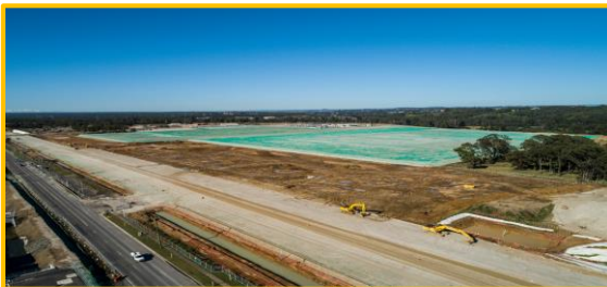
MPW precinct infrastructure works (future site of the Woolworths facilities)
