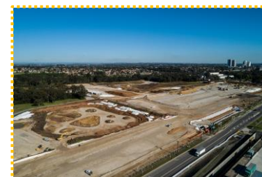
MPW precinct infrastructure works (NSW, Moorebank Logistics Park)
