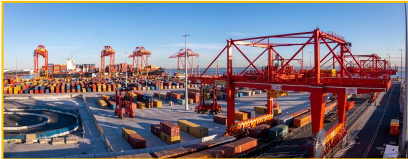
Patrick's Sydney Rail Operations now handled through the automated AutoRail terminal.
