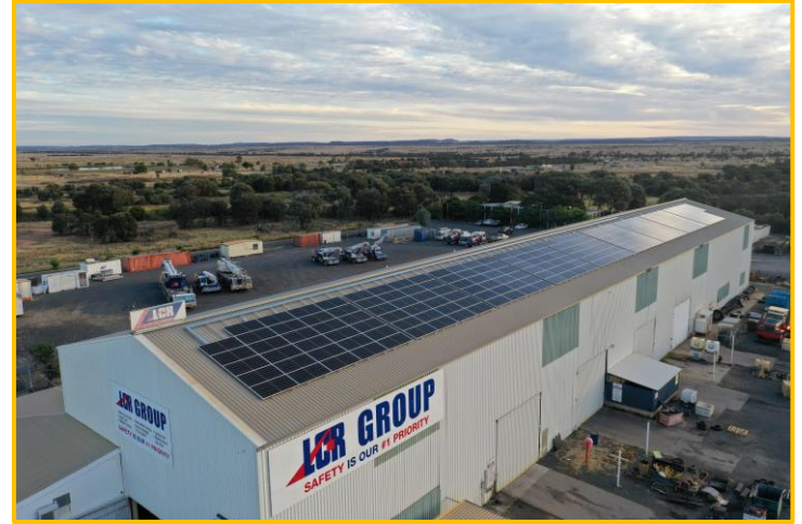
Qube (LCR) facility, Blackwater
